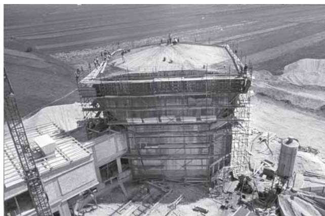
The Reactor Centre, Podgorica, built in 1966
